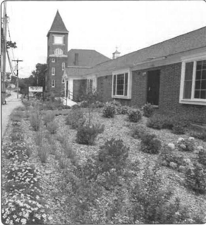
New landscaping adds the finishing touch to the Harvey-Mitchell Memorial Library expansion.
